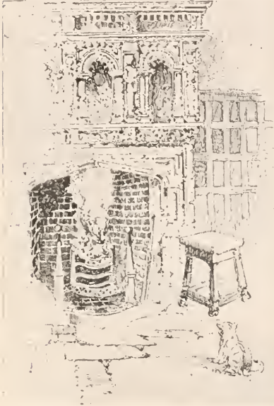
FIREPLACE IN THE LARGE ROOM, ABBOTT'S HOSPITAL.
